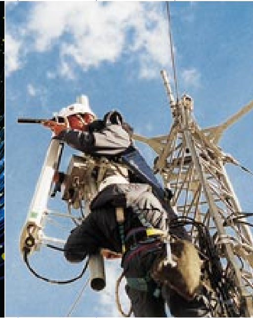
▲ Installation of an SFR antenna
