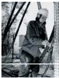
Installing radio-communication sites for Bouygues Telecom in northern Burgundy
